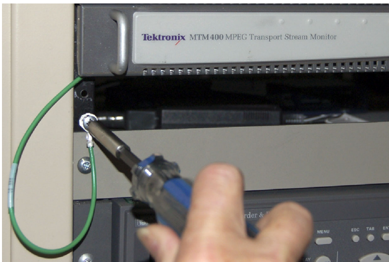
Attaching the ground strap to the equipment rack (MTM400 monitor shown)
