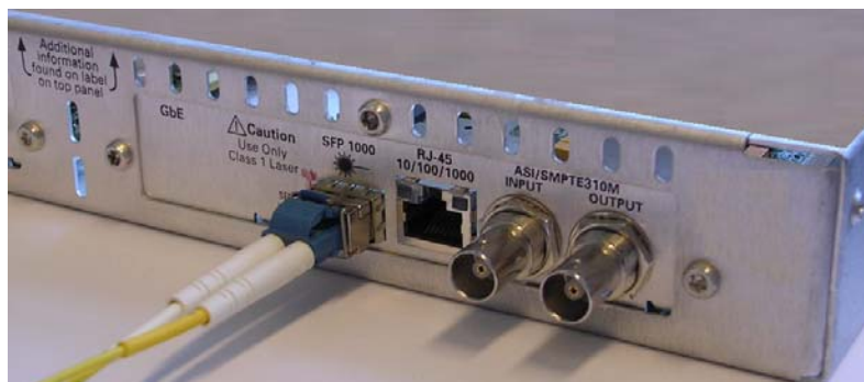
Figure 49: Optical cable connected to SFP module
