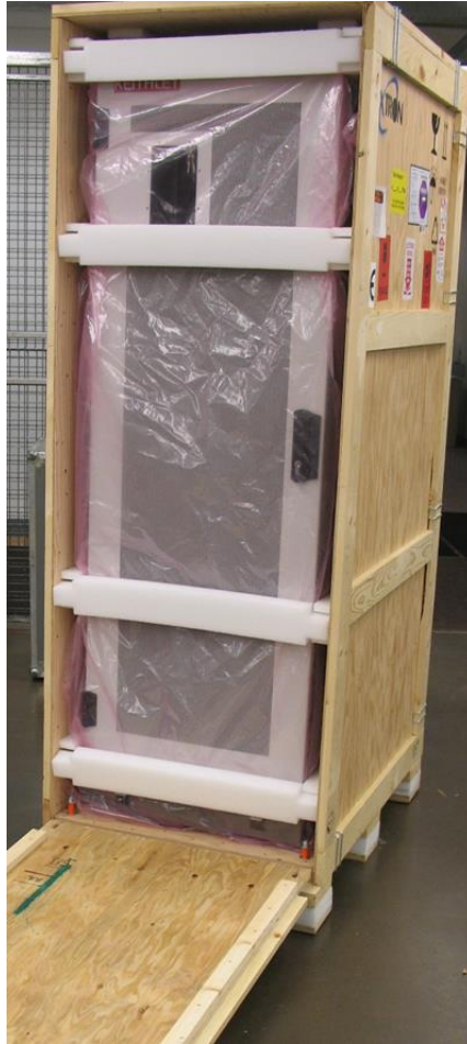
Figure 7: Removing the padding
