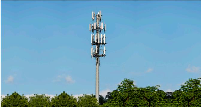
FIGURE 12. Cell Tower Using Co-Located Antenna Systems.
