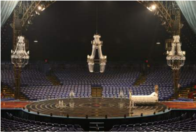
A wider view of the Cirque du Soleil Corteo stage shows the clean lines achieved by avoiding electrical wiring, while still providing a sophisticated light show. Traditional wired control is used for conventional lighting on trusses overhead and elsewhere. Wireless lighting on the mobile pieces seamlessly integrate into the overall design.
