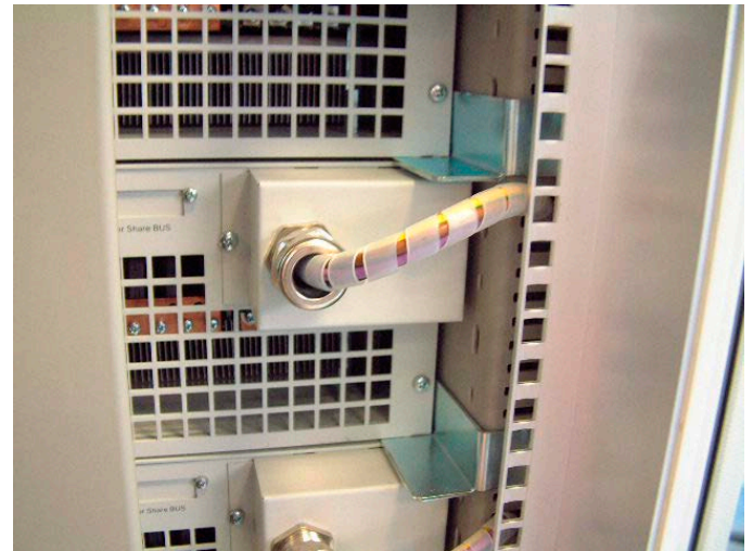
Figure 1: AC input connection of the single units
