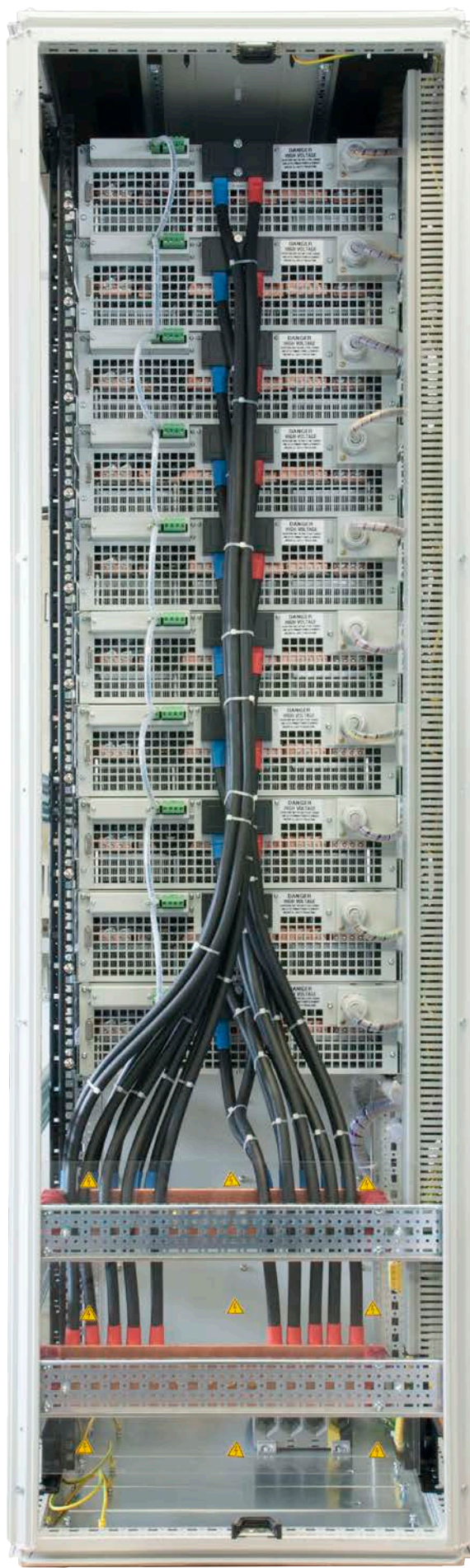
Figure 5: Rear view (doors detached)
